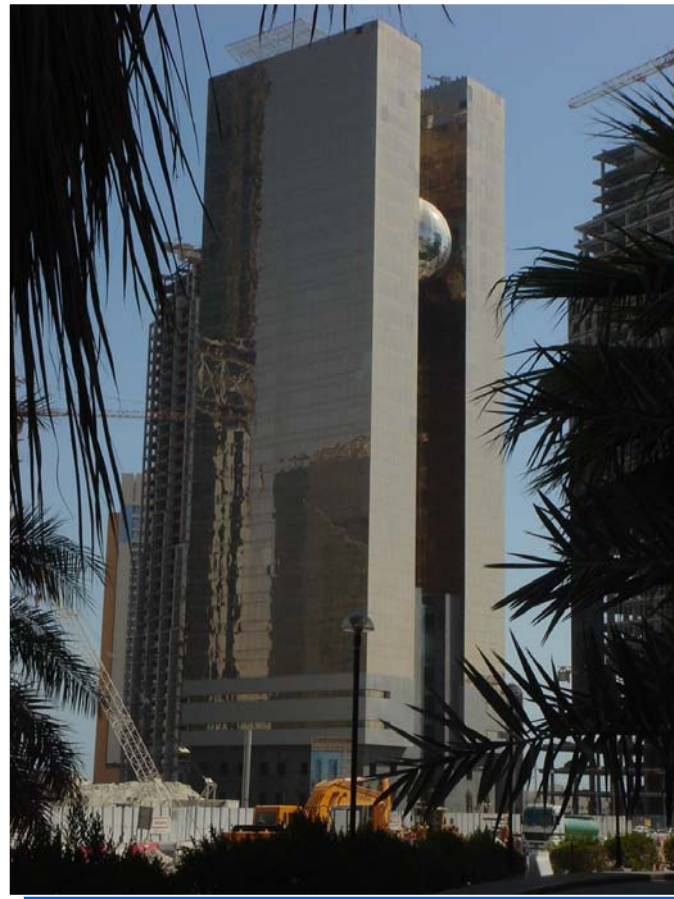
AL DANA TOWER
