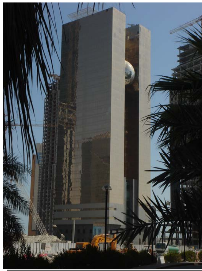
AL DANA TOWER
